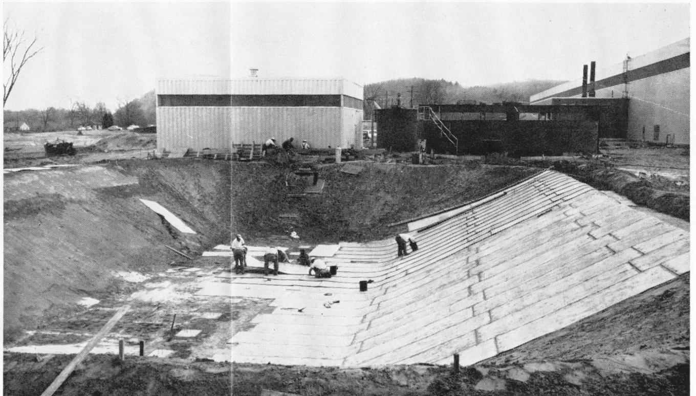
Taken during early summer, last year, this picture shows workmen laying down strips of Hydromat lining in the 120 x 75 ft. hole which now is the Equalizing Lagoon
